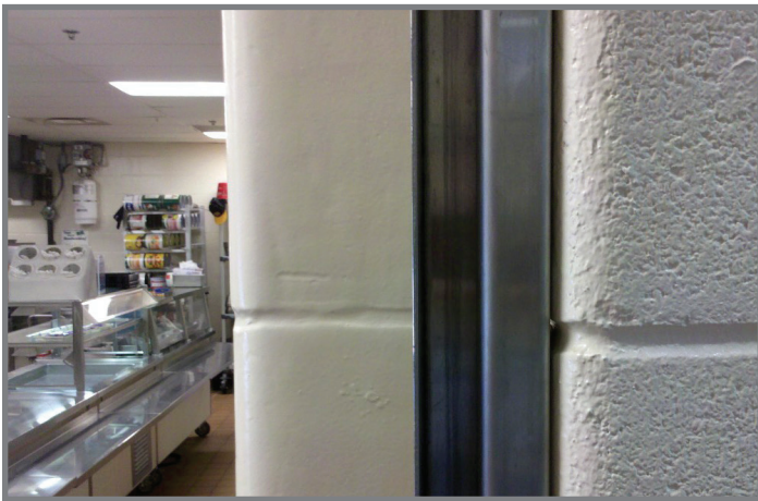
Spec-Finish Level III vs. Coated Regular Block The combination of high performance coatings and Spec-Finish block provides a pin-hole free, easily cleaned, durable smooth surface
